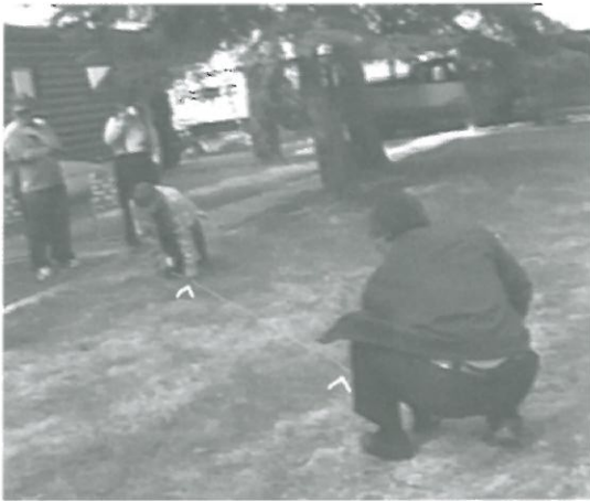
Rechecking the diagonal distance. Arrows indicate the corners.
