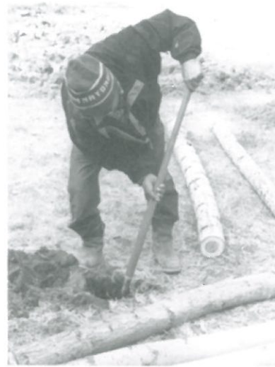
Digging the holes for the posts.
