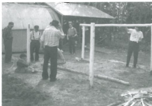
Fig. 5.10: Putting in the posts and beams for the fish rack
