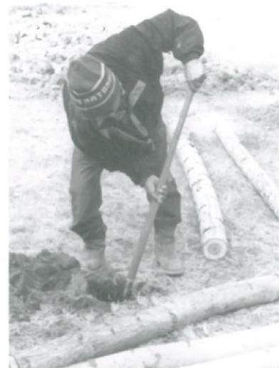
Fig. 5.9: Digging the holes for the posts
