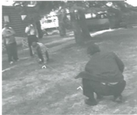
Fig. 5.8: Rechecking the diagonal distance. Arrows indicate the corners
