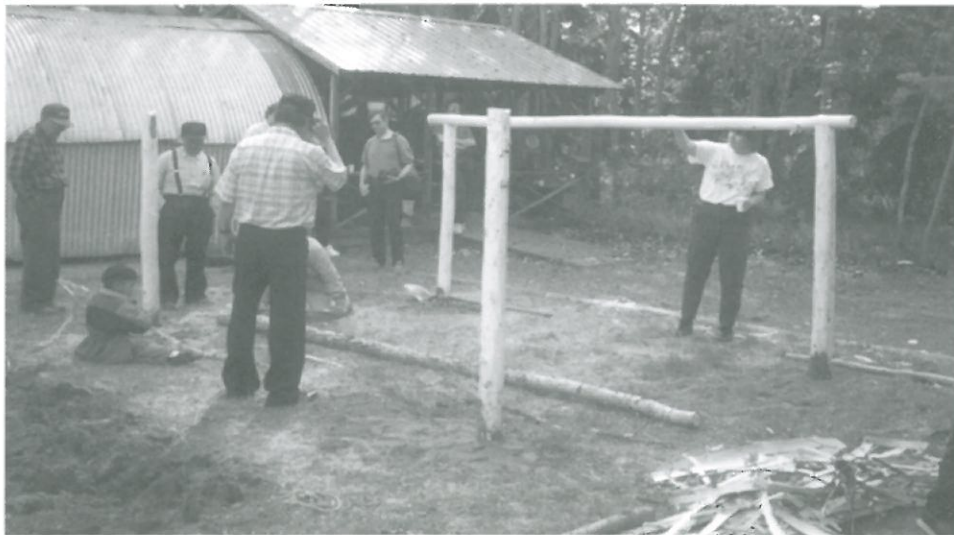
Putting in the posts and beams for the fish rack.
