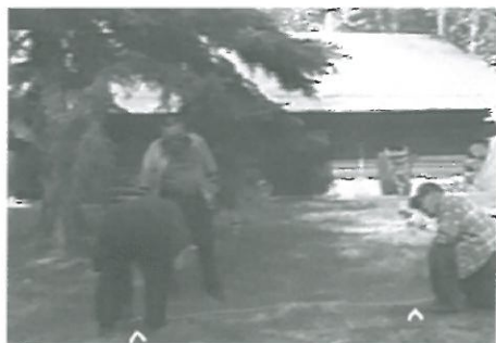
Fig. 5.6: Elders use a rope to determine the width. Arrows indicate the corners of the future fish rack
